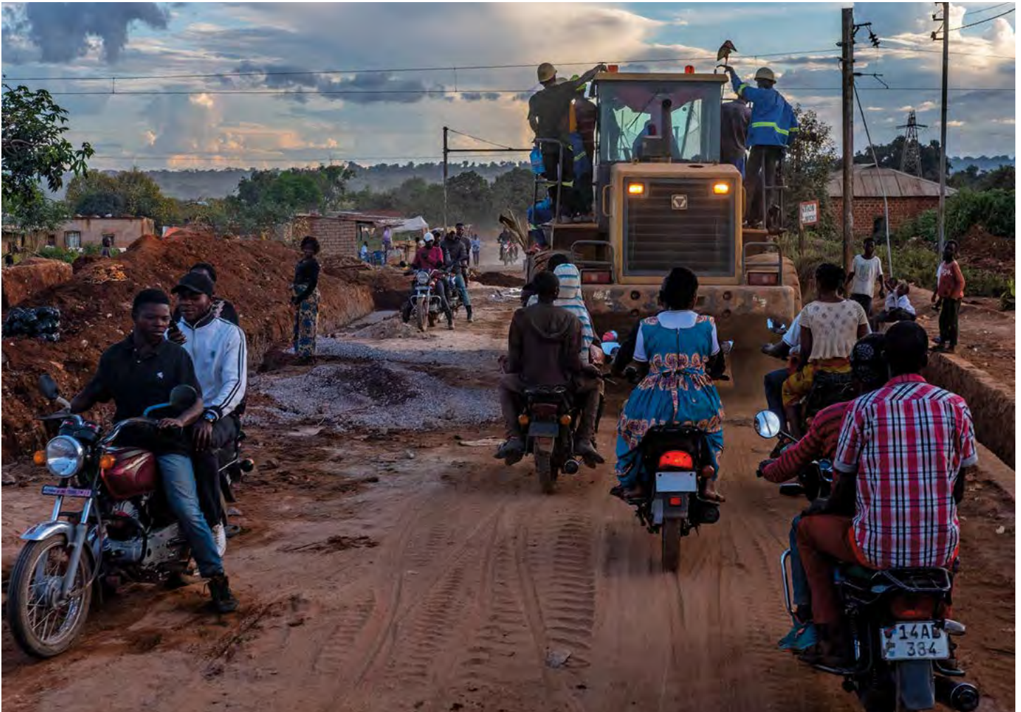
People and machinery move along a road rebuilt by a Chinese contractor near the Tenke Fungurume mine, in southeastern Democratic Republic of the Congo, on April 29, 2021. Most African countries face acute infrastructure shortages that challenge mining and mineral processing development. (Photo by Ashley Gilbertson/New York Times)
